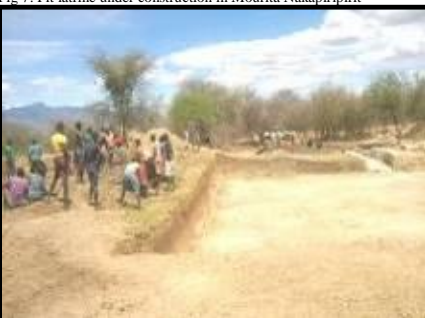
Fig 8: CFW beneficiaries during the excavation of Alakas Water Pond
