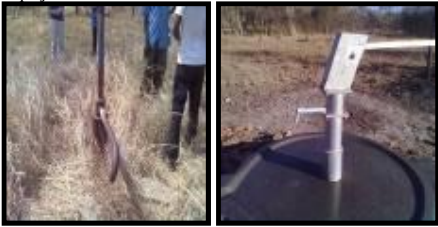
Fig5 Nanyoi Angiminito colonial Borehole: before (left) and after (right) the rehabilitation
