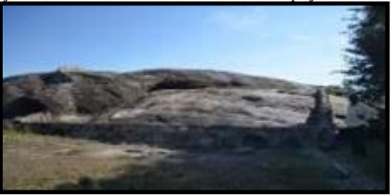
Fig 2.Rock Catchment rehabilitated under the project
