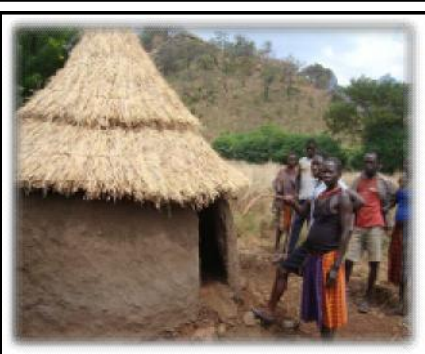
Fig 7: Pit latrine under construction in Mourita Nakapiripirit
